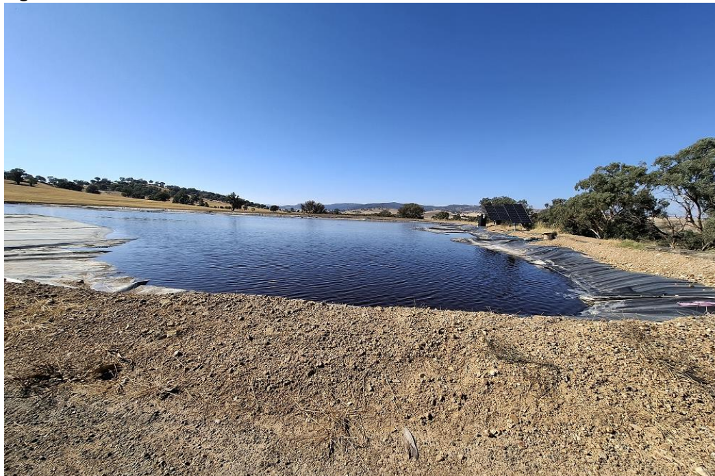
Figure 8 – Photo –Leachate Dam
